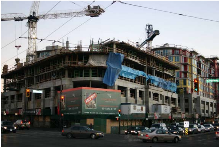
The King Edward under construction at Kingsway and Knight Street
